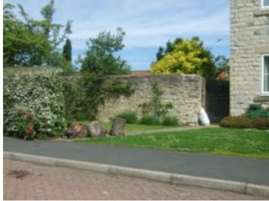
Above: Historic boundary walls near Bell's Court are proposed as the new Conservation Area b
